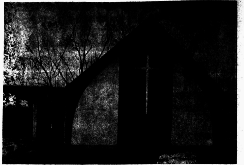
Dedicatory services for St. John's Episcopal Church will be held sometime in mid-December with the Rev. Theodore Barth, Bishop of the Diocese of Tennessee, officiating. Services are already being held at the church, construction of which was recently completed.
